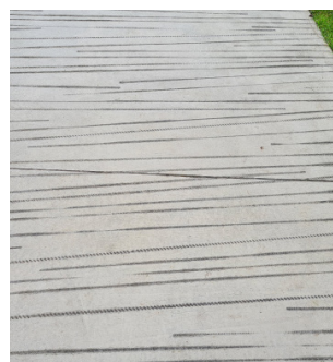
Imprinted finish in-situ concrete.
