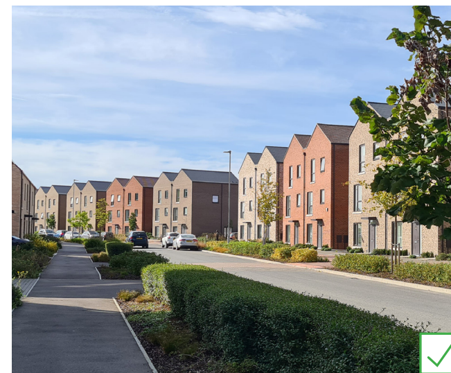
Appropriately sized verges allow for quality landscaping
