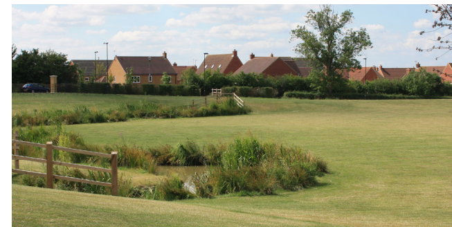
Dry basins can have multiple functions and should be well maintained
